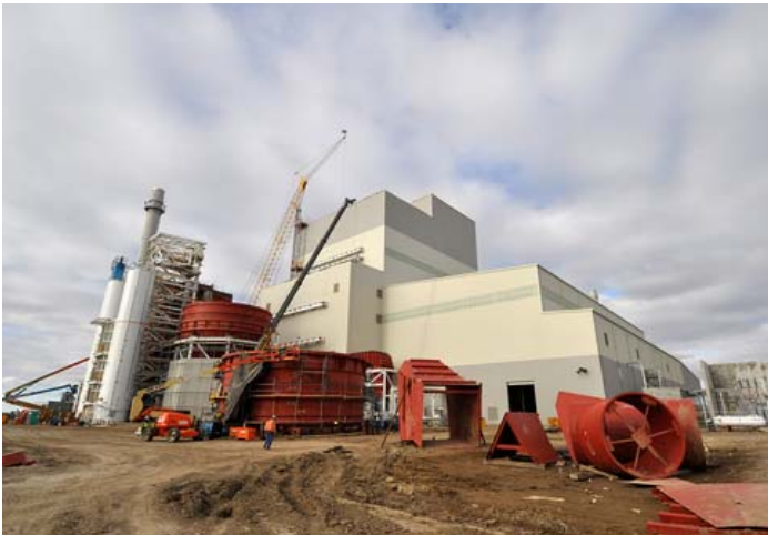
This photo shows construction of Spiritwood Station the spring of 2010.
