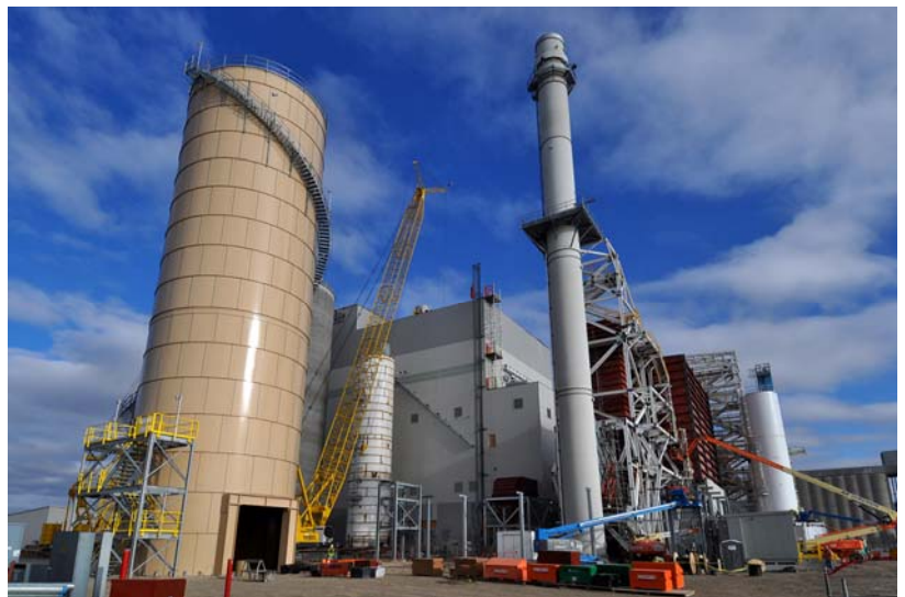
Construction of Spiritwood Station the spring of 2010.
